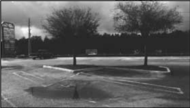
▲ Parking lot inlets are direct connections for pollutants to stormwater systems.
