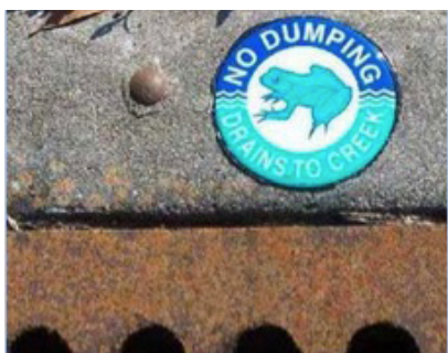
Figure 1. A “No Dumping—Drains to Creek” drain marker can inform or remind residents and guests of the drain’s direct connection to backyard waterways.
